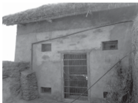
Zero Energy cellar structure for orange storage in Raikot, Jaubari, Nawalparasi
